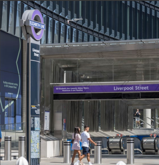
Liverpool Street Elizabeth Line Entrance
